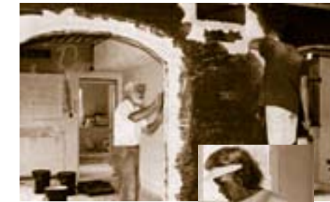
The Kreitzer family working on the walls inside the new WAS-H building.
